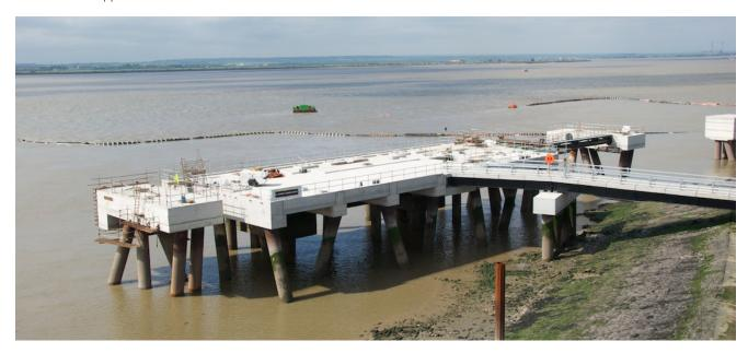
As part of the London Gateway Port development the existing bitumen and aviation fuel import jetties were demolished and replaced by a new jetty at the eastern end of the site. The new facilities are capable of taken a large range of vessels, from small bitumen carriers with less than 7,000 DWT up to large aviation fuel vessels with circa 130,000 DWT.
